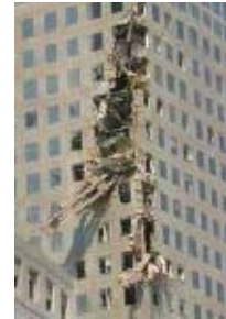
Fig. 1. Impaled Columns in Aftermath
