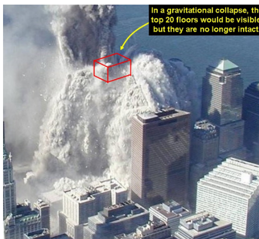
Fig. 3. North Tower Destruction –Aerial View (WTC7 is in the middle, right of center)
